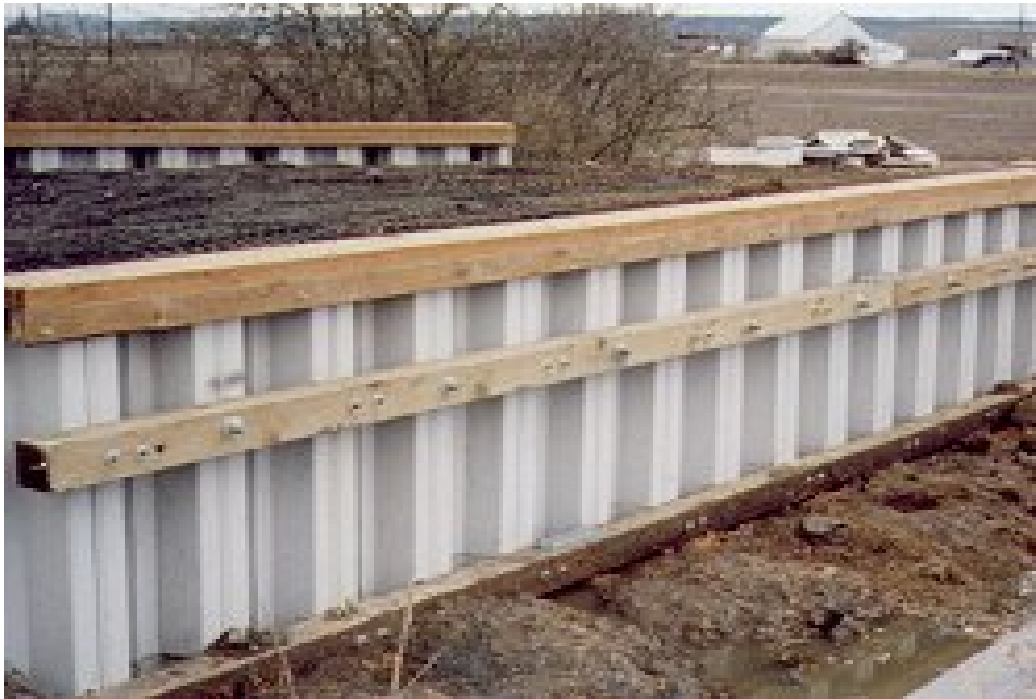
Anchored sheet pile walls
